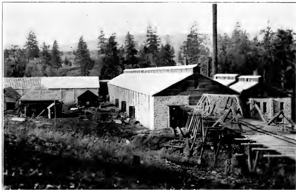
Cement-works under Construction at East Princeton.
